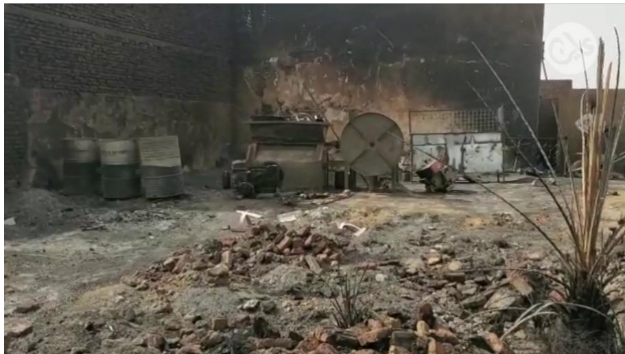
Destruction in El Fasher, Ayin
