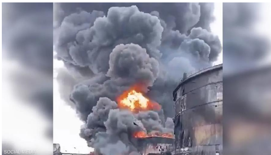
Fire at Al Jaili Refinery (Social Media)
